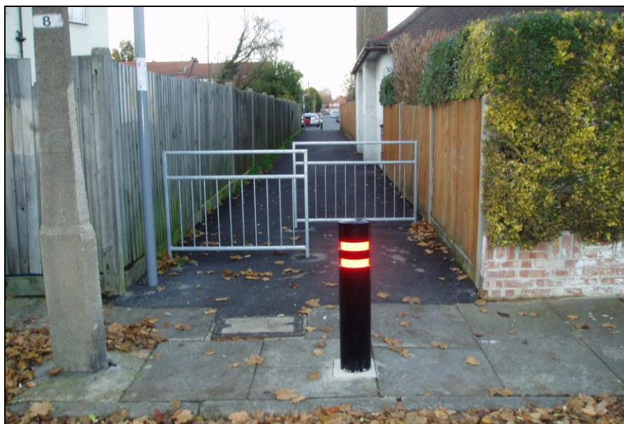
Barriers placed at footpath R174, Cranley Drive, Ruislip
