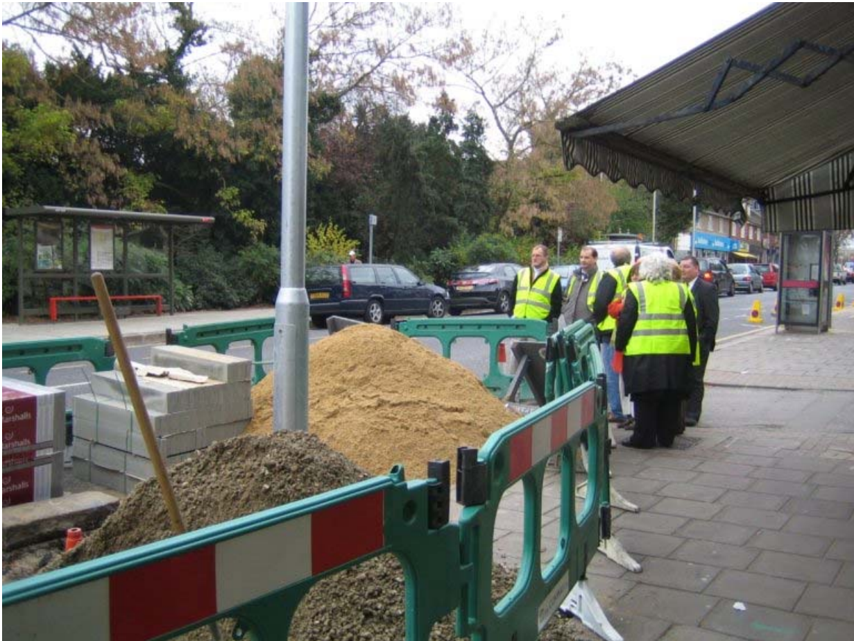
Town centre regeneration - Year 2 works in the High Street, Ruislip.
