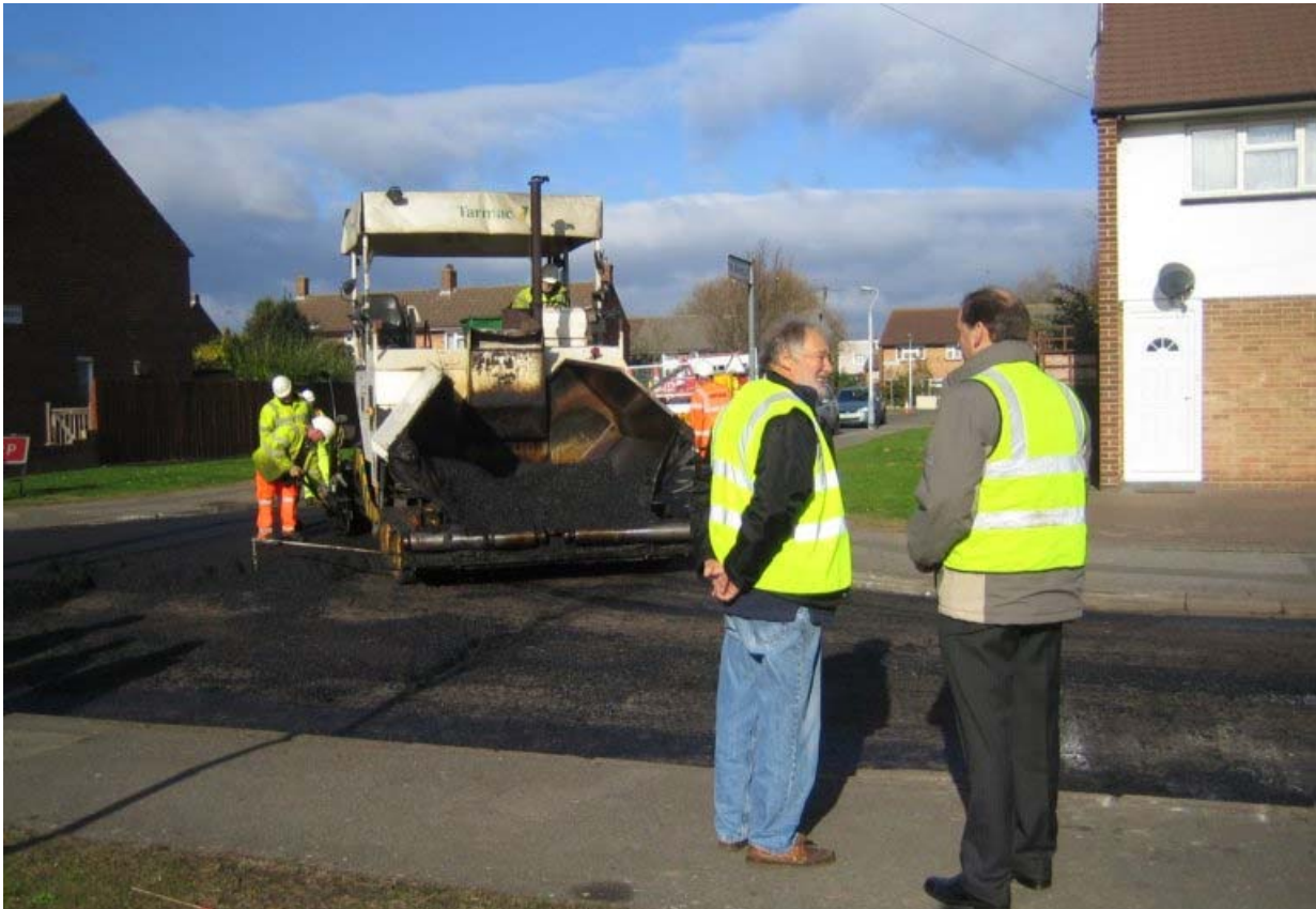
Carriageway resurfacing of The Brambles, West Drayton.
