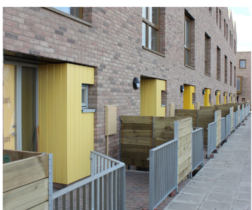
Small Windows / Timber Door
