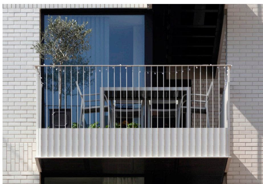
Open Metal Railings
