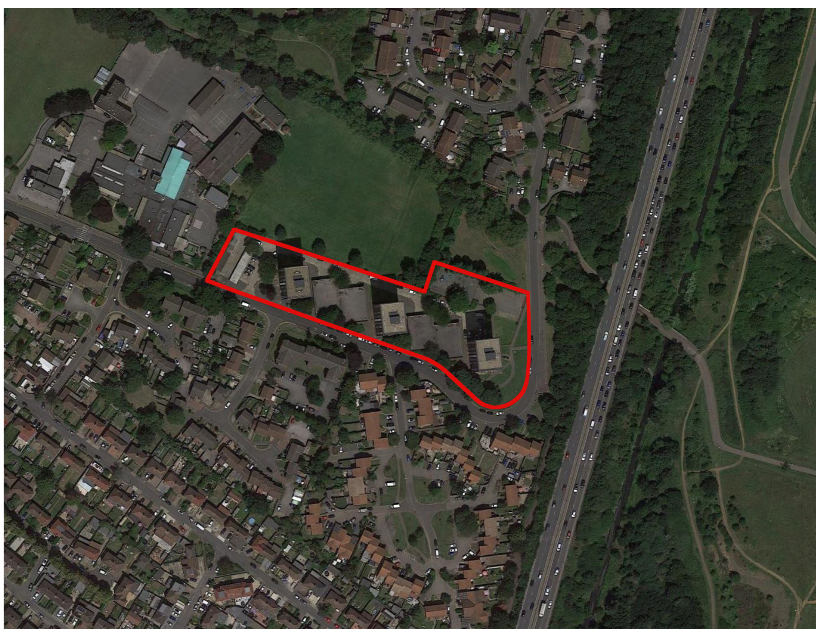
Aerial view of Avondale Drive Estate
