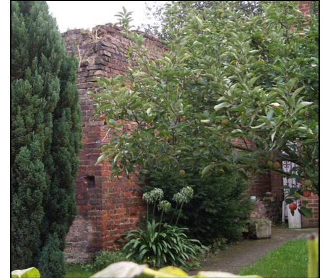
Examples of the wall types within the Conservation Area
