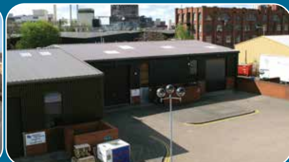
Front view of units 7, 8 and 9
