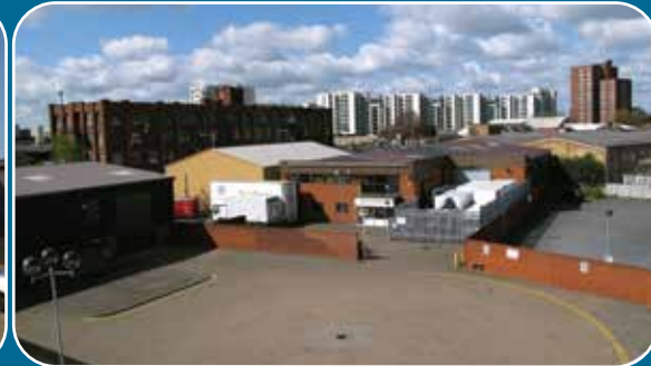
Turning area and front of unit 10
