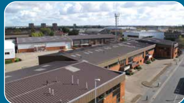
Aerial view from Silverdale road
