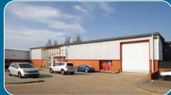
Loading area to the rear of unit 1
