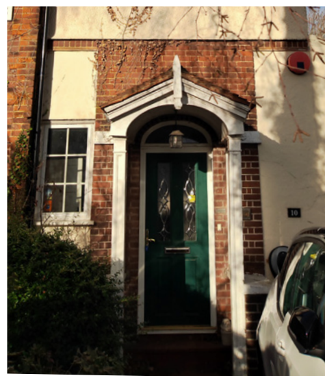
28 & 30 Morford Way – Front canopy with brackets
