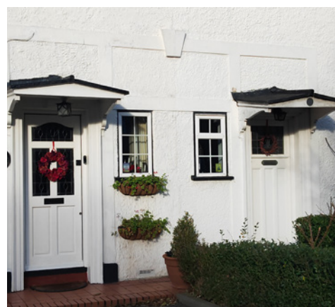
28 & 30 Morford Way – Front canopy with brackets
