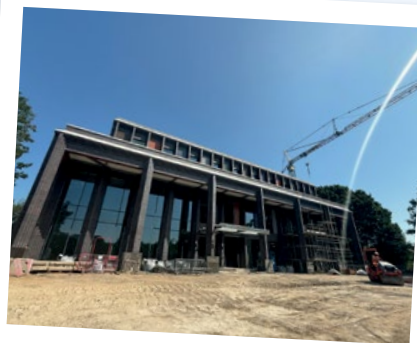
Work is progressing on the Platinum Jubilee Leisure Centre, West Drayton
