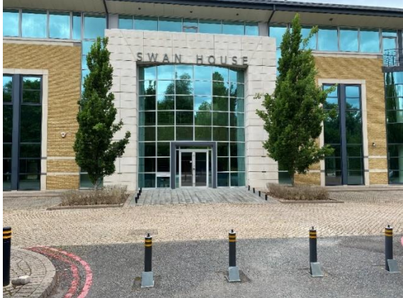
High quality office unit - vacant
