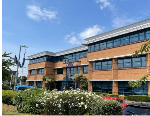
Office unit within site
