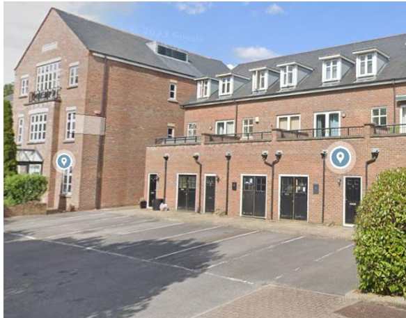
Office units within site
