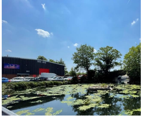
Wharf within site
