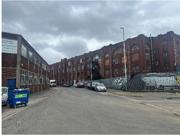
'Dirty' site environment
