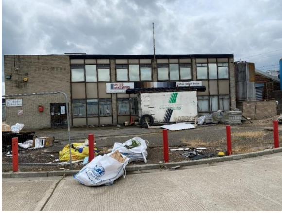
Poor environment across parts of site
