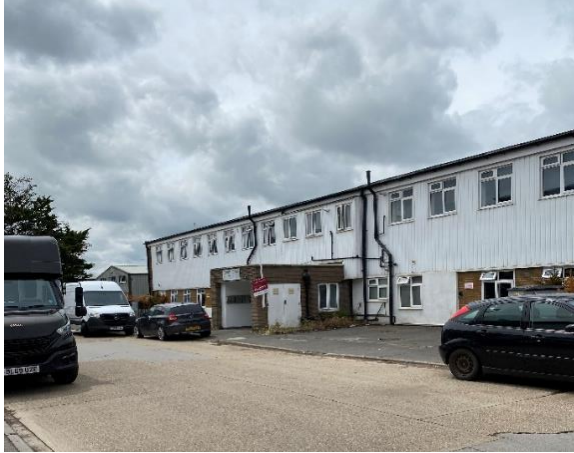
Commercial converted to residential
