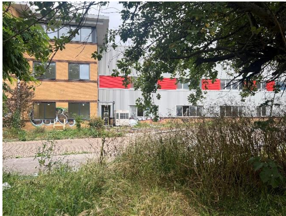
Refurbishment of Pasadena Centre
