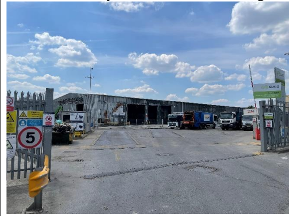
Suez waste facility (re-build after fire damage)
