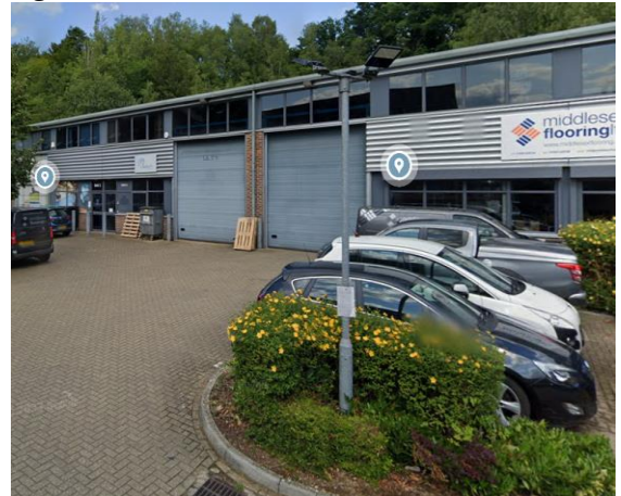
Light industrial units within site
