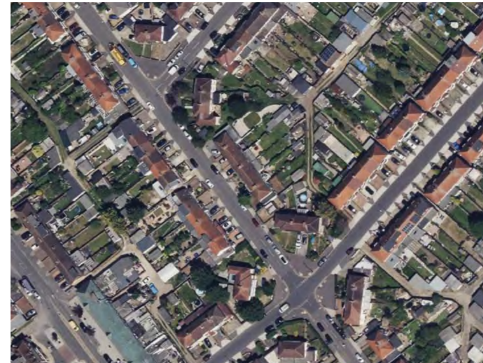
Aerial View, Ryefield Avenue, Uxbridge © Bing Maps
