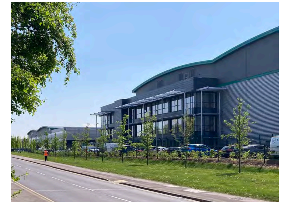
Virtus Data Centre, Horton Road, Hayes © Hillingdon Council
