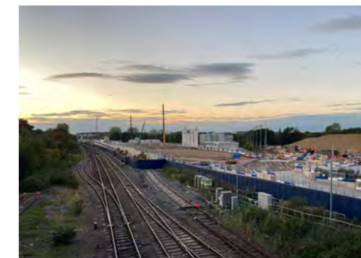
View from Long Lane towards HS2 construction site, Ickenham © Hillingdon Council
