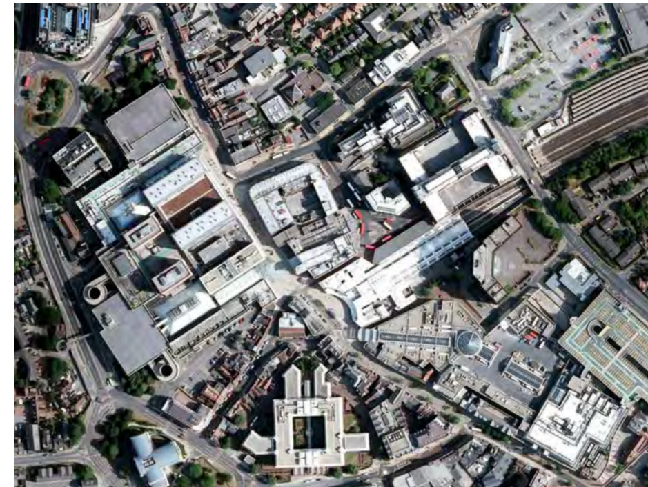
Aerial View, Uxbridge Station © Google Maps
