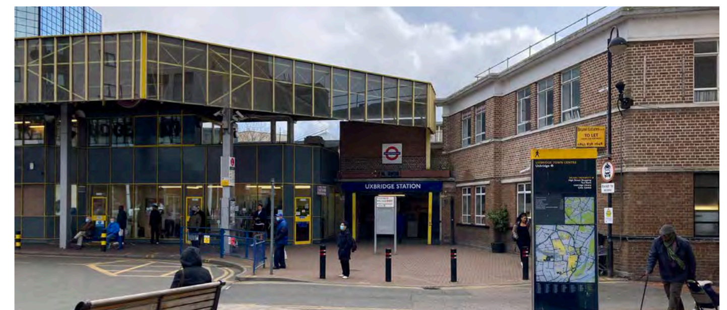
Uxbridge Bus/Tube interchange seen from Bakers Road © Hillingdon Council 2022
