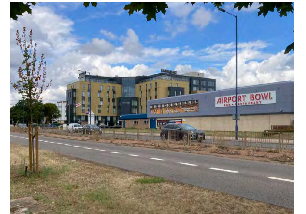
Airport Bowl, Bath Road, Harlington © Hillingdon Council
