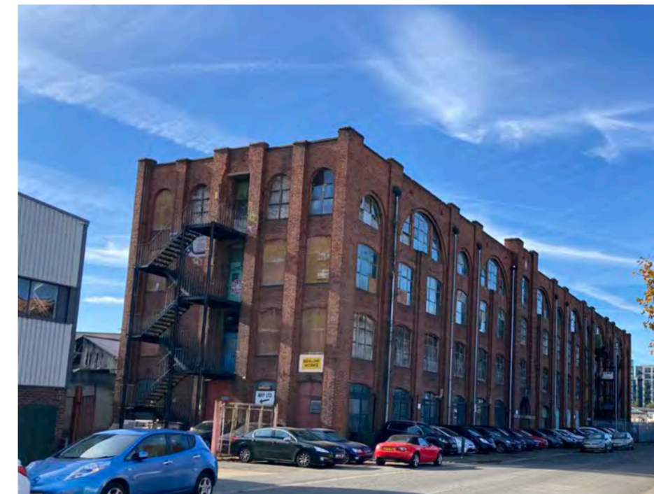
Benlow Works, Silverdale Road, Hayes © Hillingdon Council
