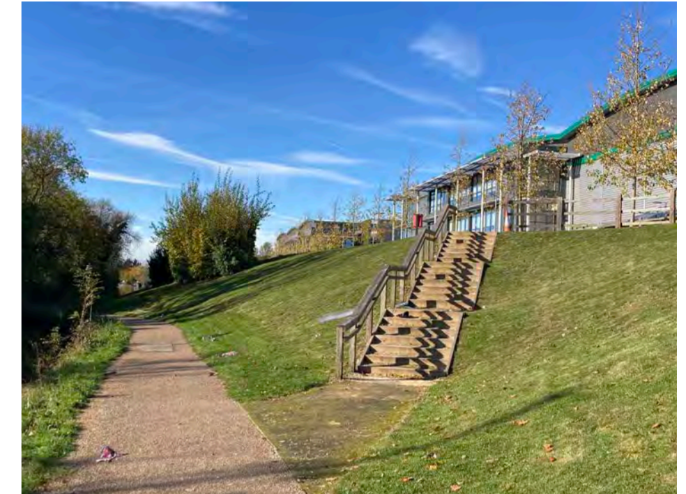
Data Centre, Grand Union Canal, Hayes © HC
