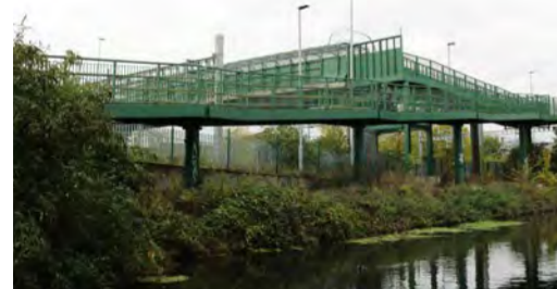
West Drayton, Cycle Route over railway © Hillingdon Council
