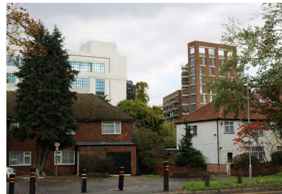
Tall building behind terraced housing, Hayes © HC
