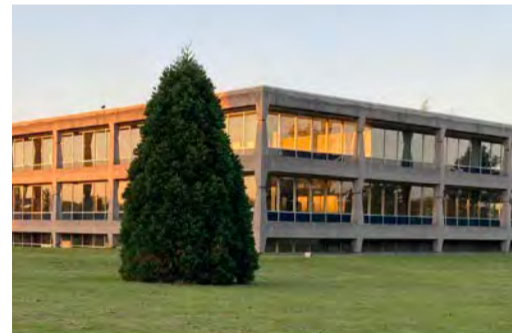
Former Heinz Headquarter and Research laboratories, Hayes (Grade II* listed) © Hillingdon Council
